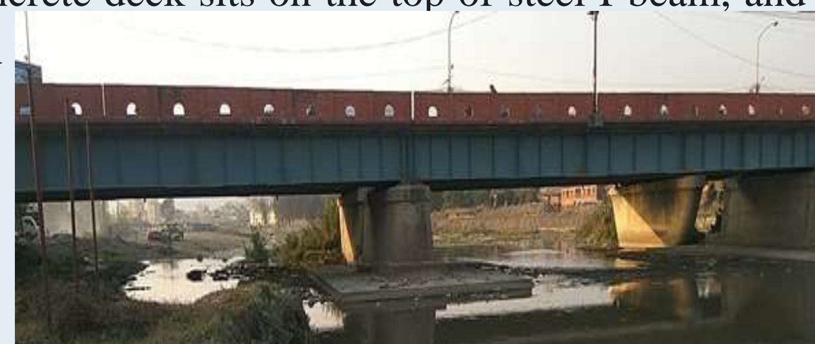
Fig. 1. A side-look of Kupondole-Thapathaly Bagmati River Bridge.
